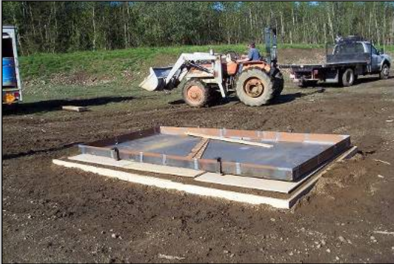
Final shot readied for detonation
