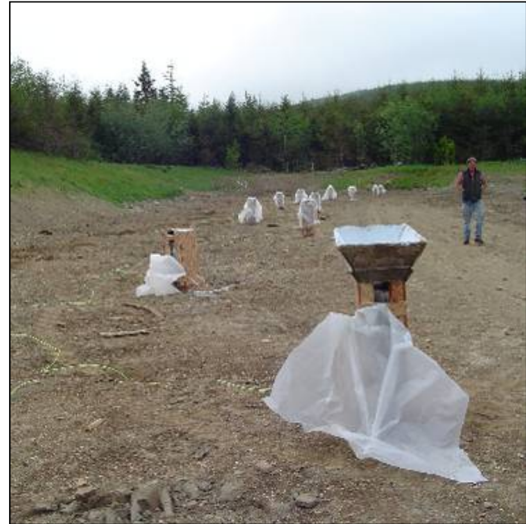
Hoppers for pouring explosives into charge gap
